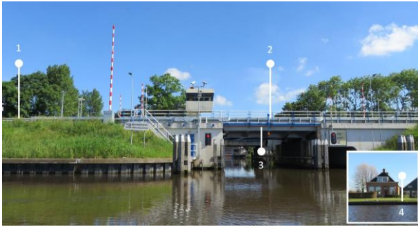
Figure 2. Overview of several measurement positions necessary to determine the bridge correction conform the measurement protocol from the National Public Works and Water Management Office (1= reference point besides the road; 2= point above the bridge; 3 = point below the bridge; 4= immission point in the direct environment)
