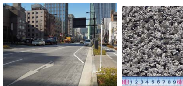
Figure 8. Condition of heat-insulating pavement
