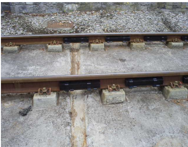
Photograph 3: Rail dampers.
