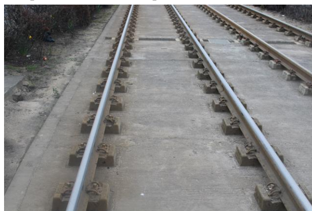
Photograph 1. Traditional slab track
