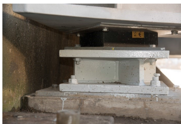
Figure 7: New rubber block support under renovated A44 bridge.
