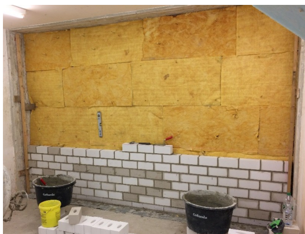
Figure 1: Construction of exterior wall in wall sound transmission facility of the HFT Stuttgart.
