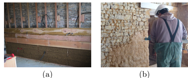
Figure 1. Different construction methods associated to hemp-concrete density: Shuttering (a) and Spraying (b). Some pictures courtesy of Vincent Corbard.
