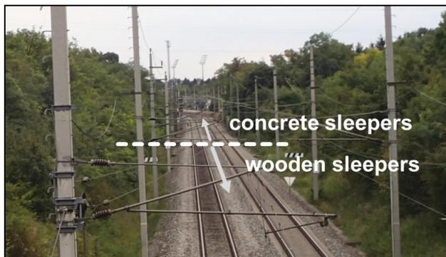
Figure 2. Test track for the estimation of the difference in emitted airborne sound depending on the sleeper type.
